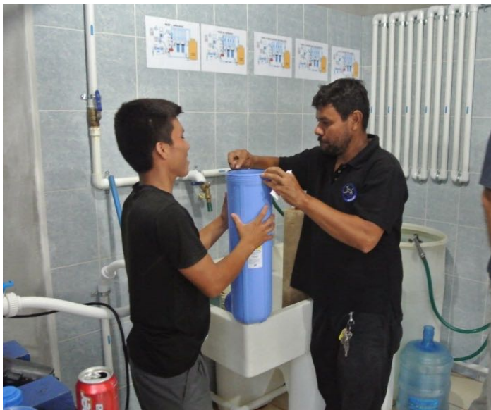
Maintenance of an existing system.
