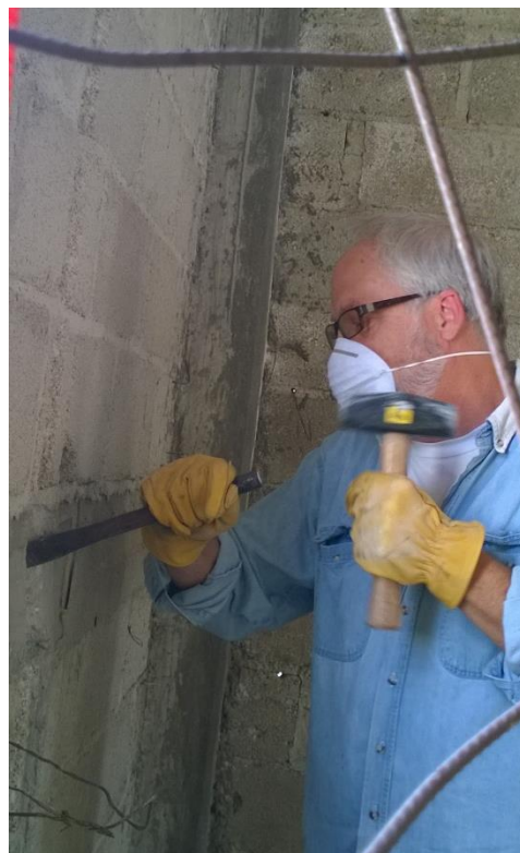
With mallet and chisel making space for a wiring conduit in Puebla
